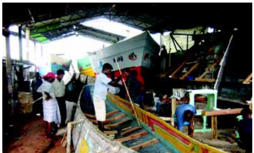
Boat replacement and repair – an important part of short-term tsunami rehabilitation.
